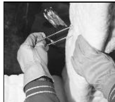
Figure 6 - Inserting Packing Pin into Batten Strip Overhead
